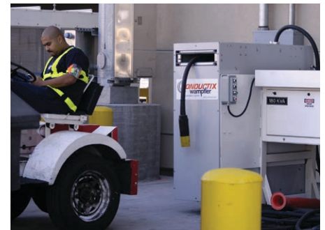
The PLB400 can be used with any model of 400 Hz converter; shown here mounted next to the converter.
