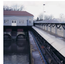
Open the gates! Program 0330 cable trolley system on a lock
